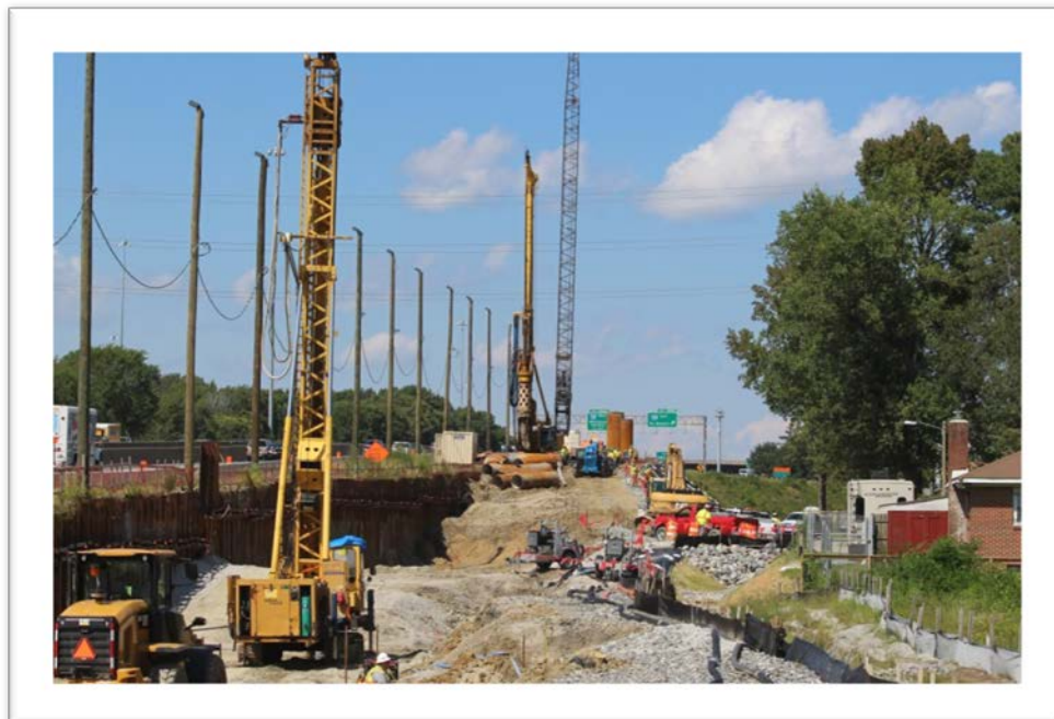
Densified Aggregate Pier Drilling (foreground) at Retaining Wall M and P (I-64W)
