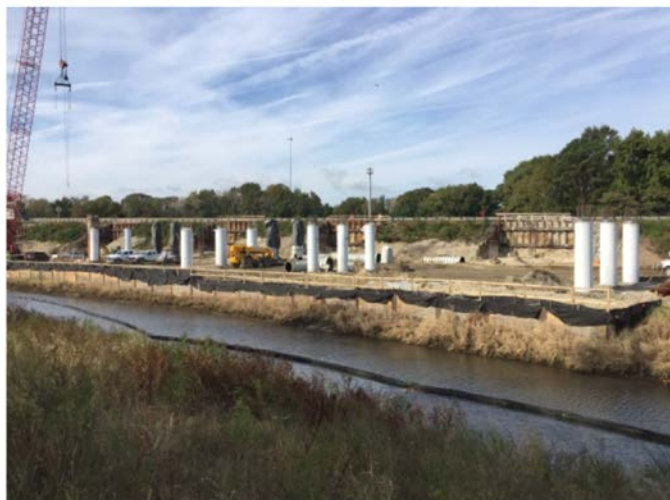
Column Construction along Tidal Channel
