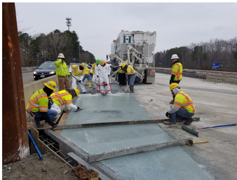
Latex Modified Concrete Overlay Placement I-64 EB over ramp to Rte. 143
