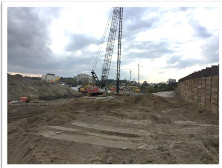
**Pile Driving Bridge B-601 with Support of Excavation Wall (right, looking west)**
