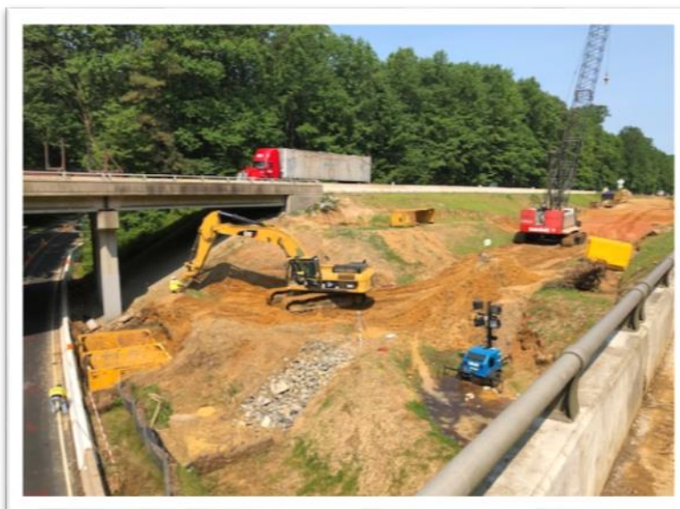
Bridge construction at the east abutment of Lakeshead Drive
