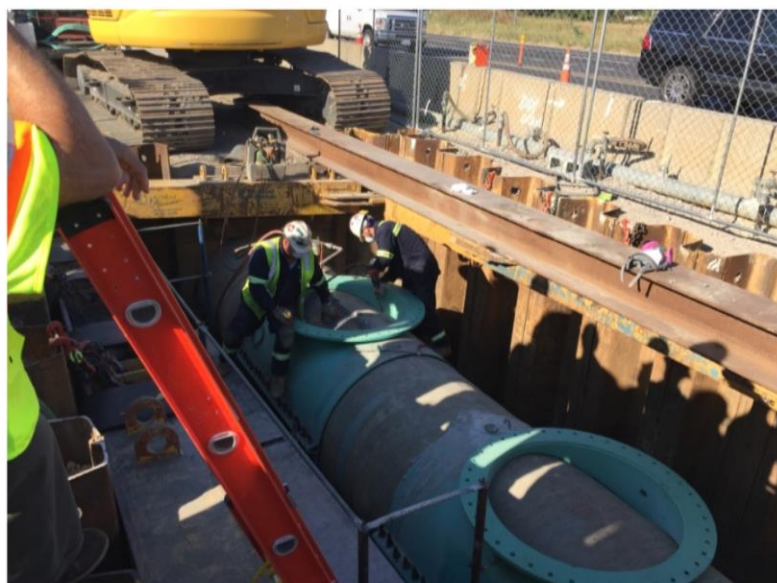
Installing Bypass Collars for 48" Diameter Force Sewer Main on Newtown Road
