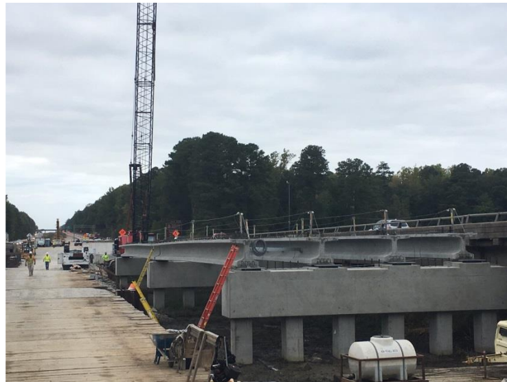
Concrete beam installation WB Queens Creek Bridge
