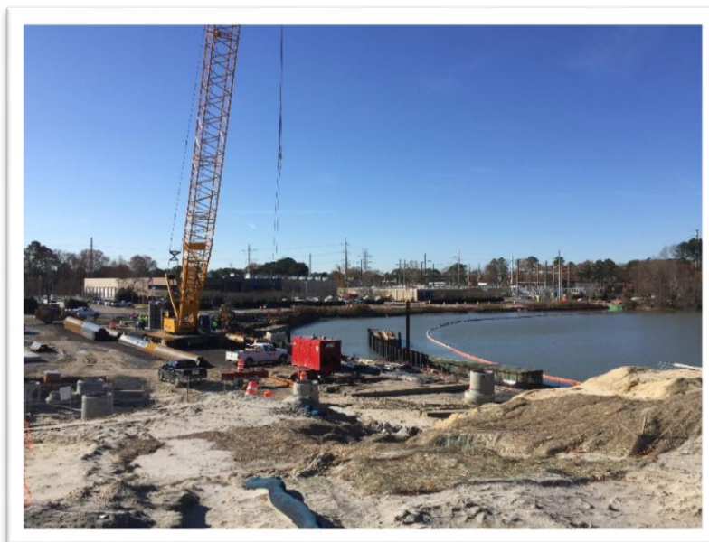
Setting Sheet Piles Bridge B-621
