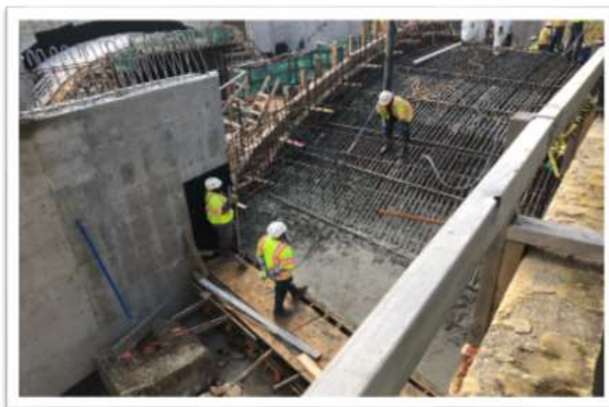
Concrete placement for the cast in place arch section of the EB I-64 bridge over the Colonial Parkway
