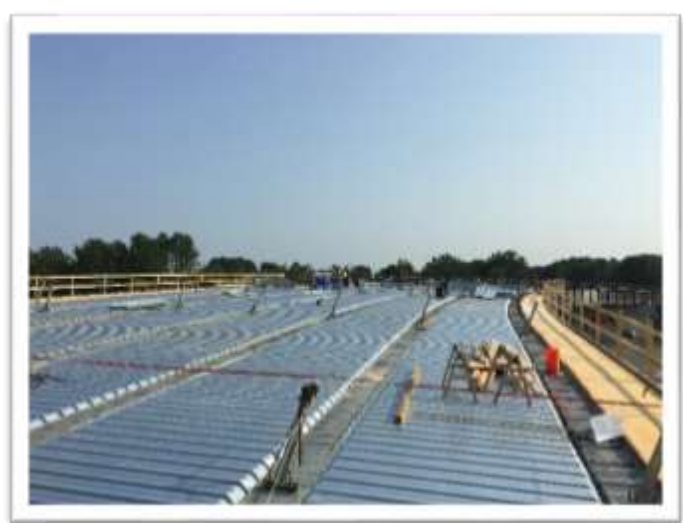
Stay in Place Forms and Overhangs on Flyover Bridge
