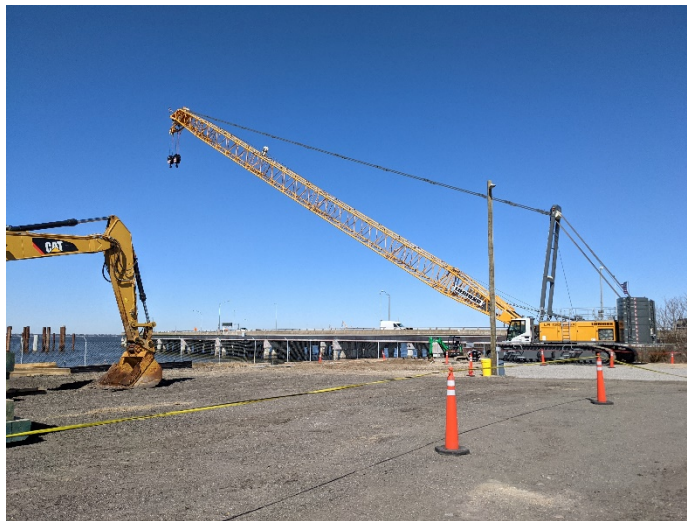
◀ Willoughby Spit Crane Mobilization for Temporary Construction Trestle
