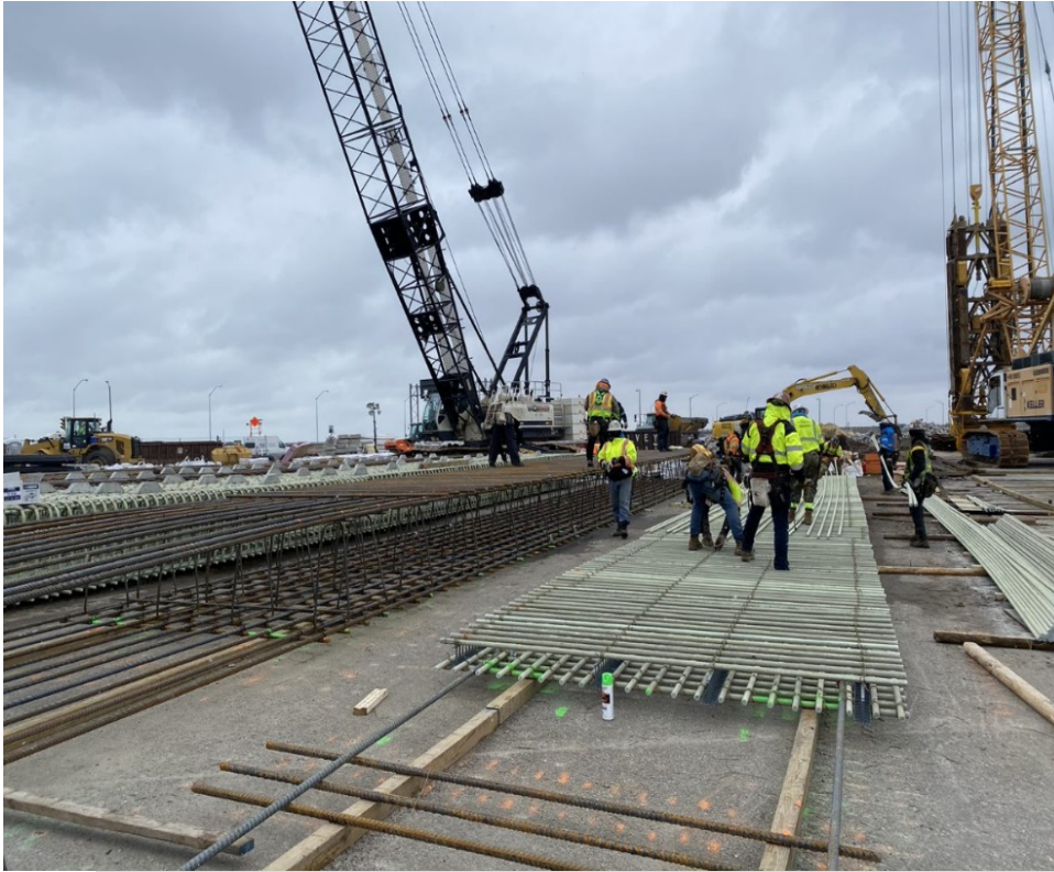
◀ South Island Slurry Wall Panel Rebar Cage Fabrication
