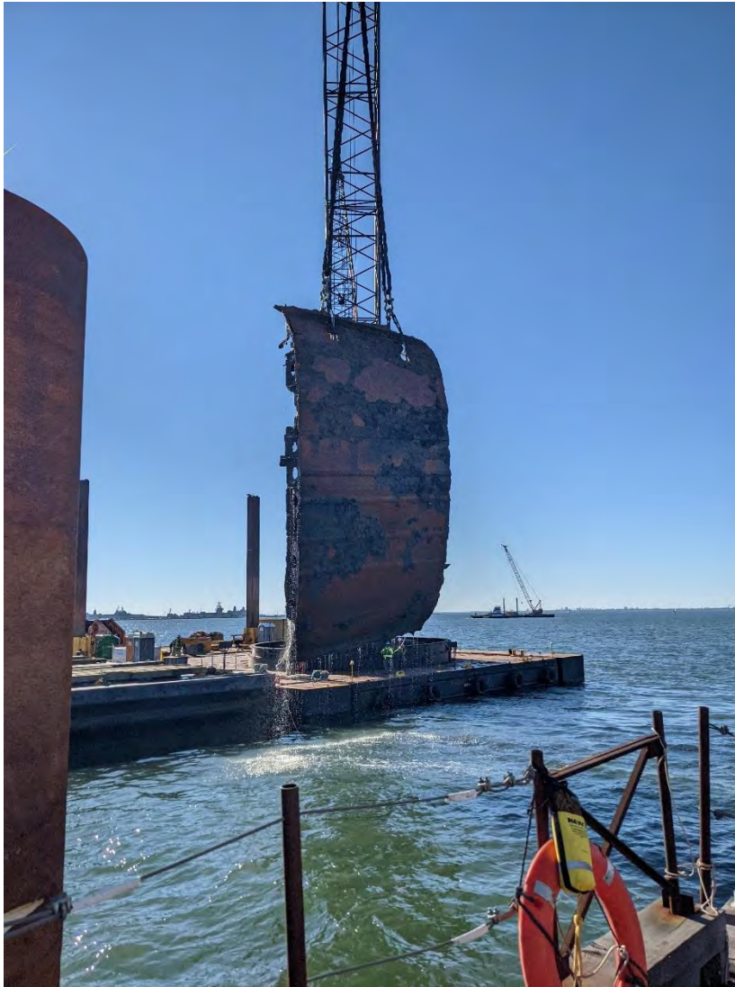
◀ South 1 Temporary Construction Trestle Removal of sunken vessel.
