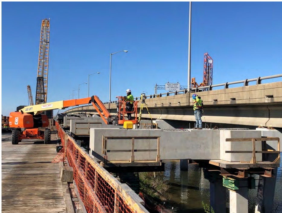
◀ Willoughby Bay Bridge Precast cap placement and survey.
