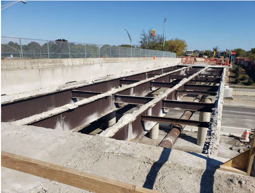
◀ Mallory St Bridge Demolition of existing bridge for future widening.
