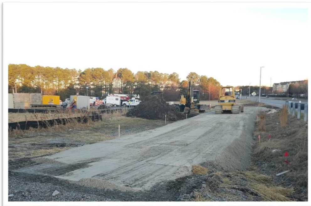
Equipment Pad at Backup Generator Site 64-104
