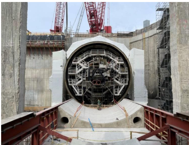
◀ South Island TBM Shield and Gantry Cradle
