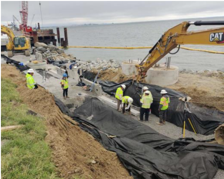
◀ Retaining Wall 108 Eastbound Panel installation near Hampton shoreline
