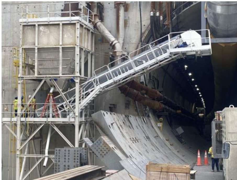
◀ South Island Assembling ballast delivery system at tunnel entrance
