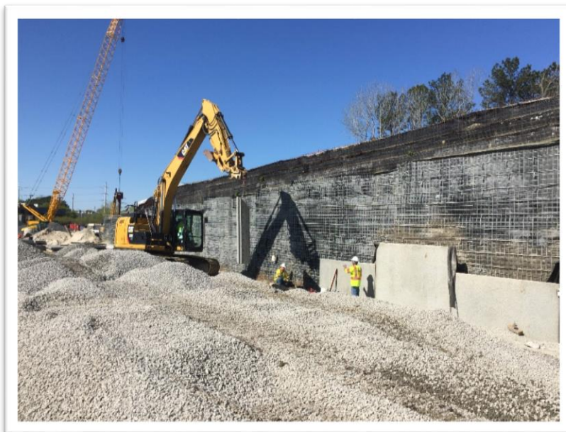
Placing Fascia Panels (typical throughout project)
