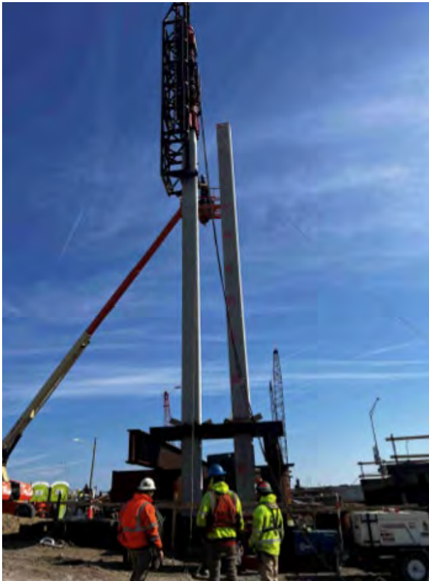
◀ South Trestle Ramp B Abutment A pile driving
