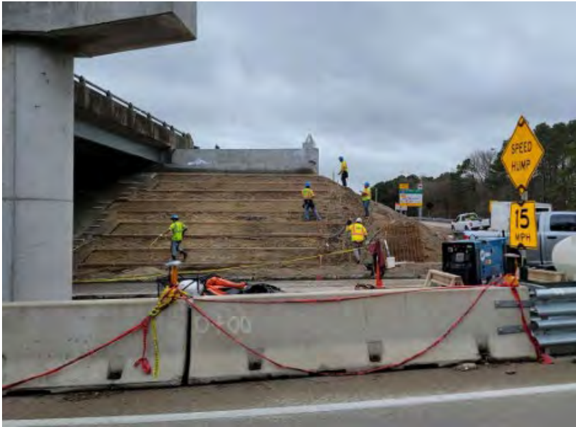
◀ Patrol Road Bridge Eastbound Abutment B slope protection work
