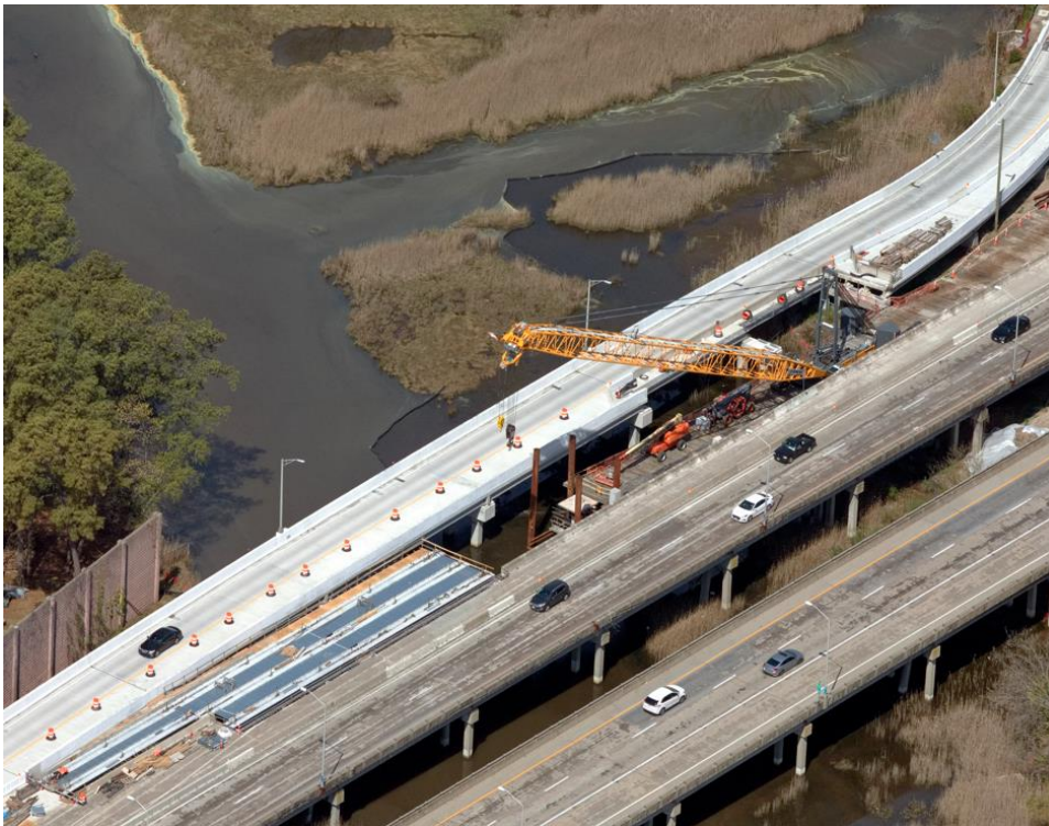
◀ Bay Avenue Bridge Eastbound Deck formwork installed between existing bridge and new ramp
