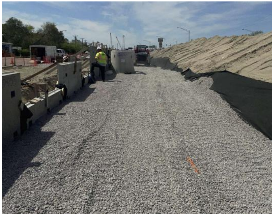
◀ Bayville Street Installation of retaining wall 302
