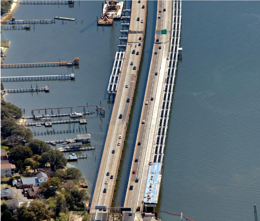
◀ Willoughby Bay Bridge Widening Eastbound girders nearly complete, progress continuing for Westbound girders
