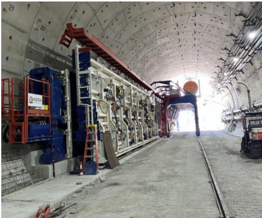
◀ HT Tunnel Egress Structure Formwork in Tunnel
