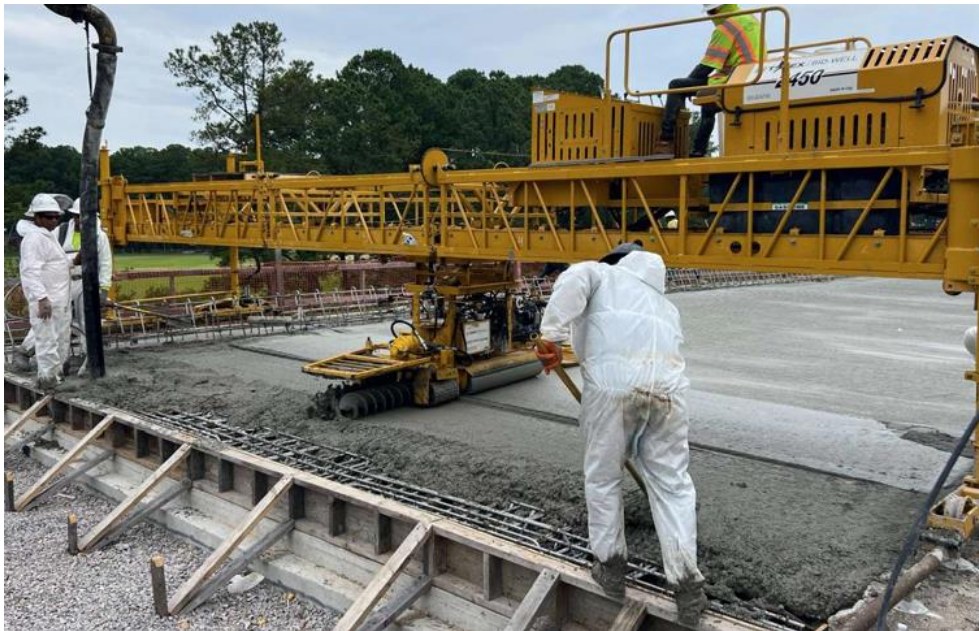
◀ Oastes Creek Bridge Eastbound Spans 17 - 18 deck concrete placed
