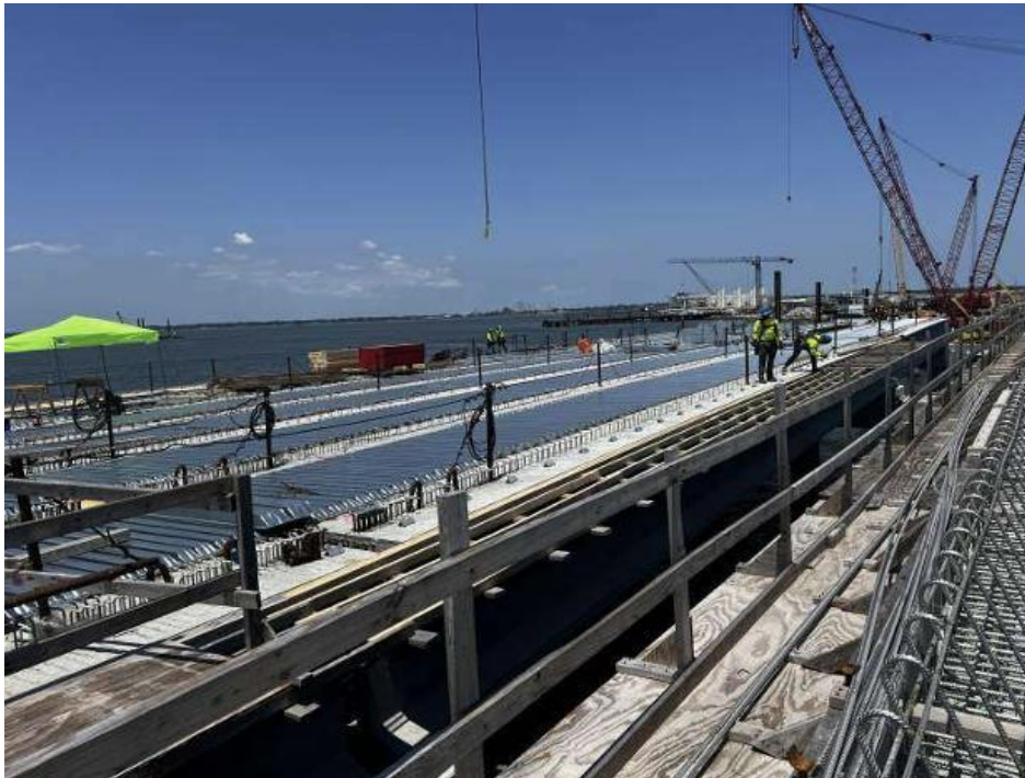
◀ South Trestle Eastbound Installation of Span 11 Stay-in- Place forms
