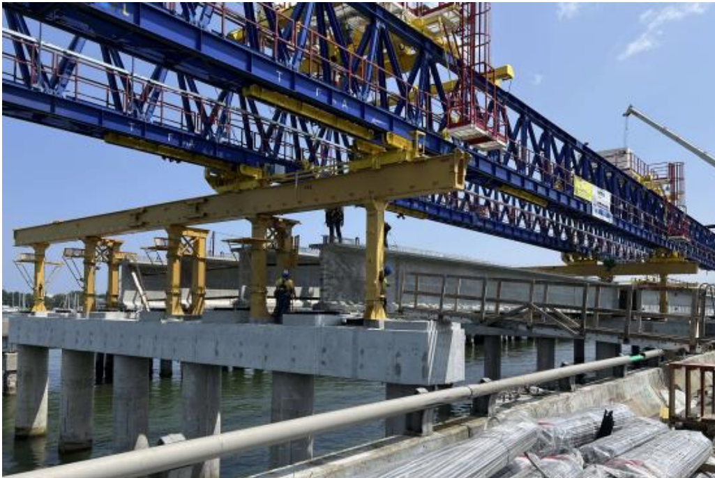
◀ North Trestle Westbound Beam Launcher installing girders at Span 23
