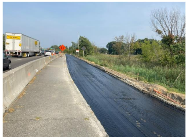
Placement of Cement Treated Aggregate I-64EB
