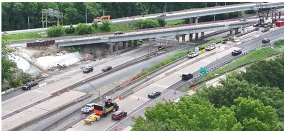
Widening of I-64-EB Bridge over I-564
