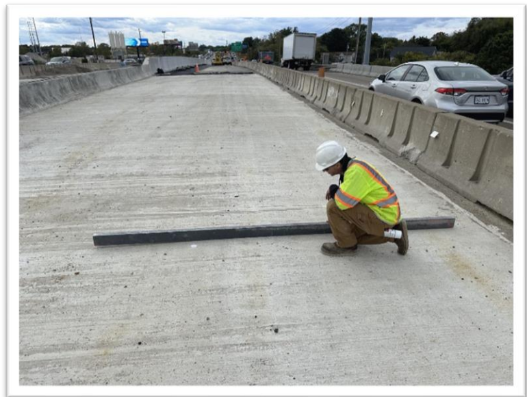
HREL 4C Quality Control Manager using 10-foot straight edge to measure bridge deck smoothness over King Street
