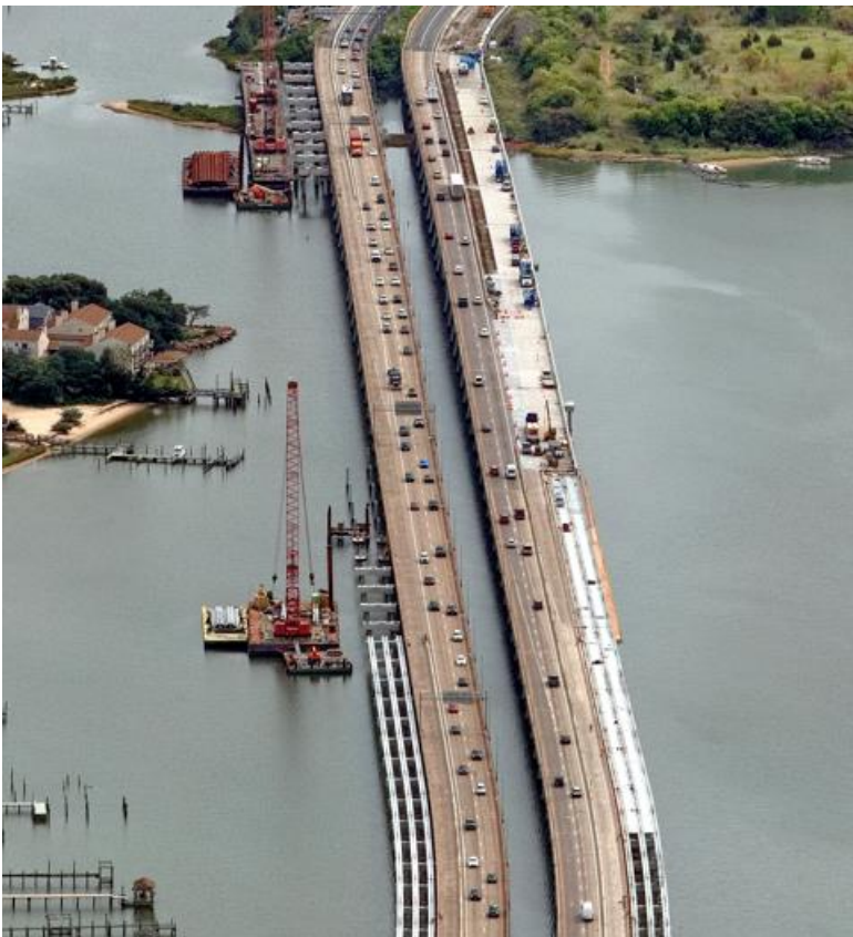
◀ Willoughby Bay Bridge Eastbound Rehabilitation and widening of bridge
