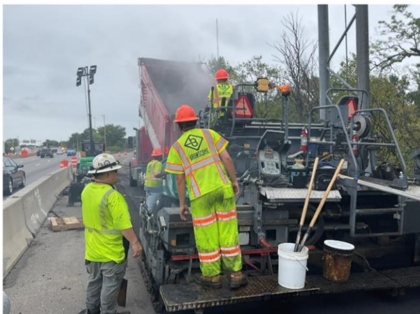
Asphalt Placement I-64 EB Outside Shoulder
