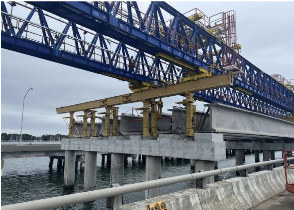
◀ North Trestle Westbound Installation of Span 20 girders
