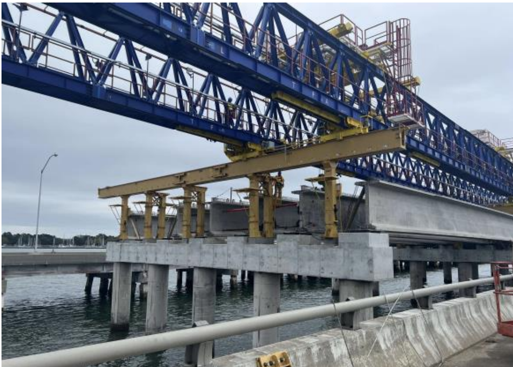
◀ North Trestle Westbound Installation of Span 20 girders
