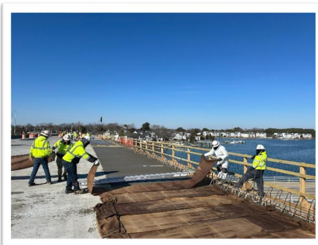
Hampton River Bridge (I-64 WB) Freshly placed concrete with wet burlap being placed for curing
