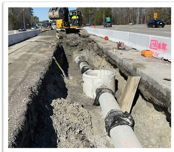
Storm Drain Installation in I-64 median
