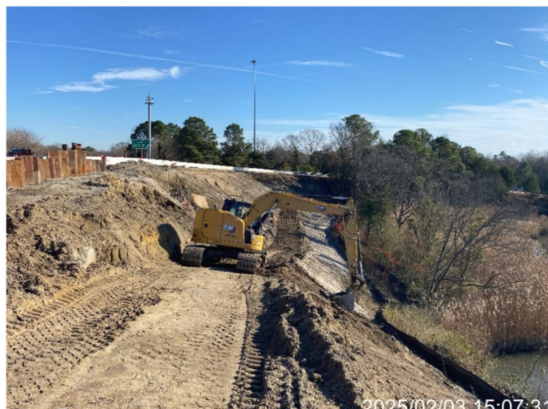
Tidewater Drive Loop B Ramp Embankment Construction
