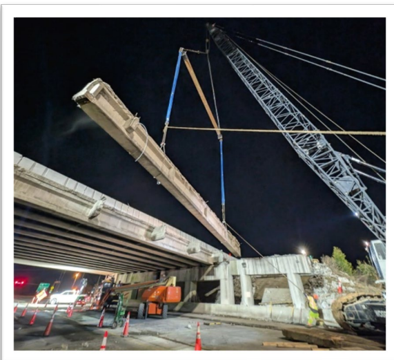
I-64 LaSalle Ave Bridge Girder Removal
