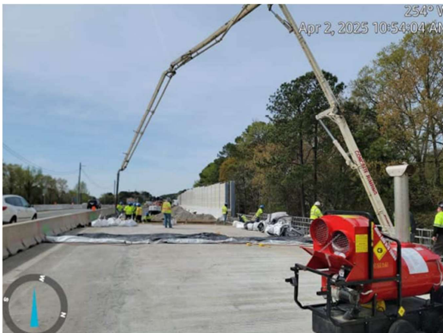
◀ Bayview Bridge Approach slab abutment B placement
