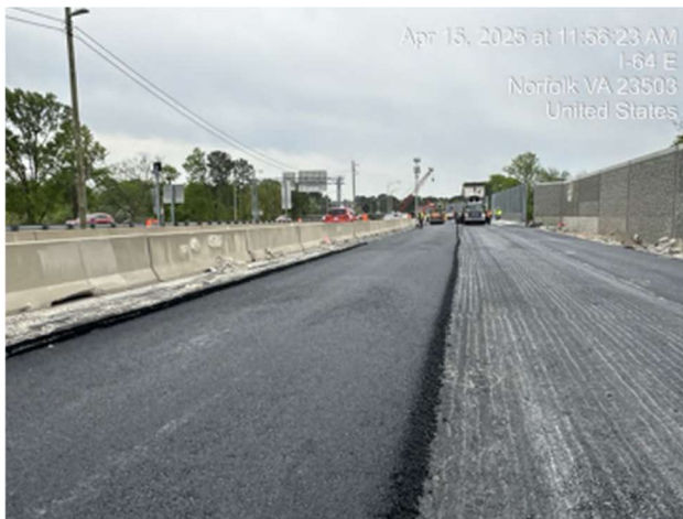
◀ Retaining Wall 402 Asphalt Placement
