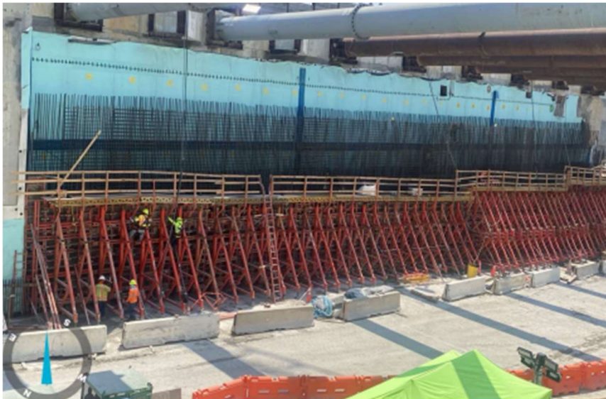
◀ North Island Cell 2 East Wall Pour 2 Reinforcing Steel Installation
