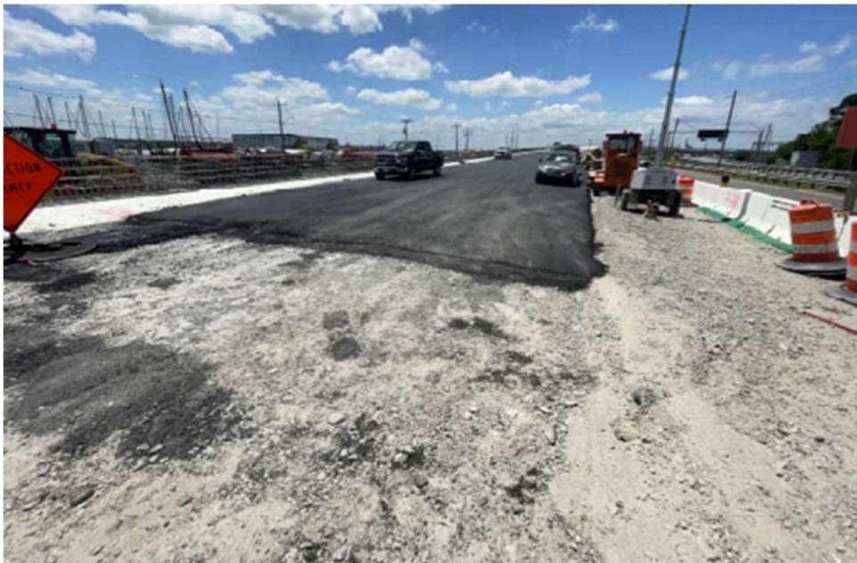
◀ Segment 3B Placement of Lift base asphalt along Retaining Wall 301
