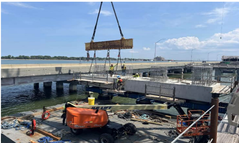
◀ North Trestle Westbound Installing Bent 7 Cap
