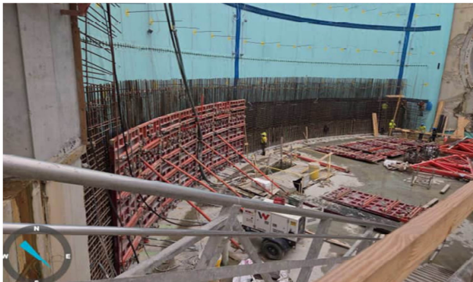
◀ North Island Cell 1 East Exterior Wall Reinforcing Steel & Formwork
