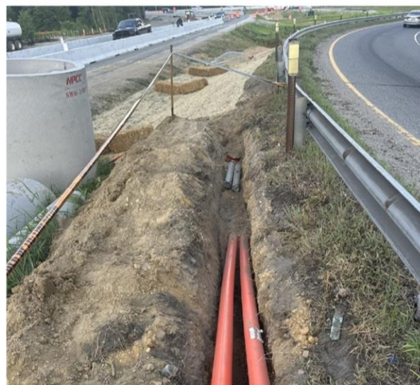
Conduit and Junction Box Installation
