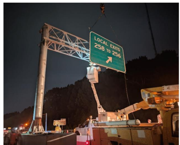
Overhead Sign Structure Installation
