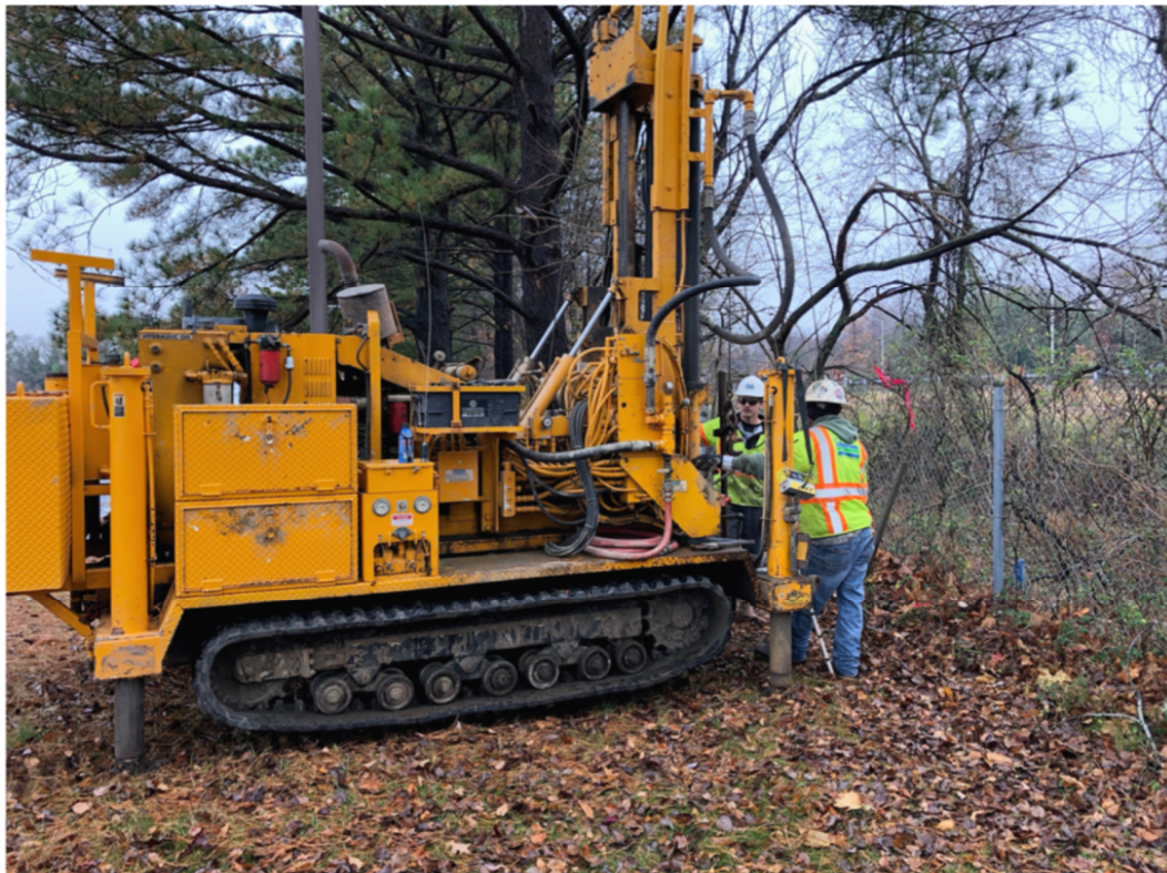
Geotechnical boring at Hampton University
