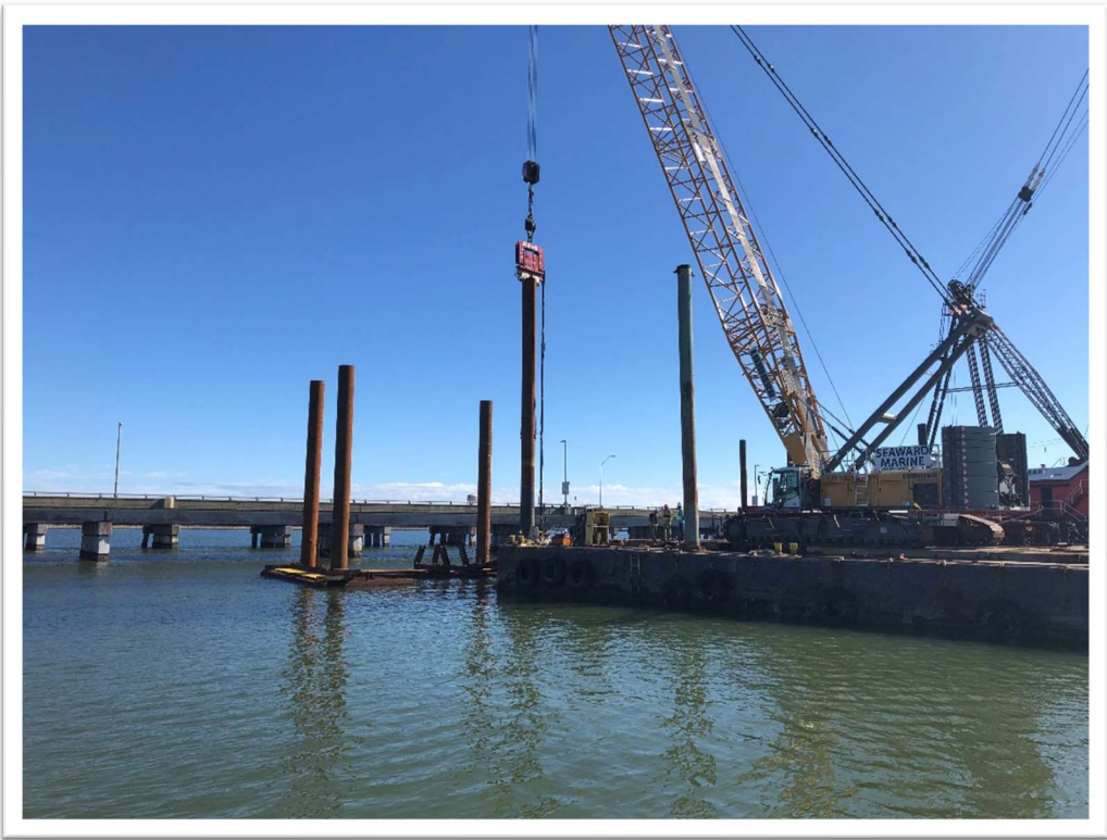
Piles for Temporary Construction Trestle N1
