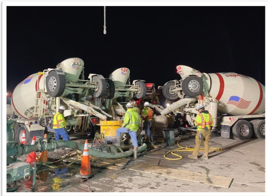
South Island Slurry Panel Concrete Placement
