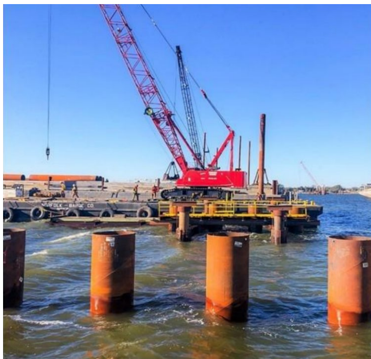
◀ North Island Expansion Pile Driving Operations performed by Seaward Marine Corporation
