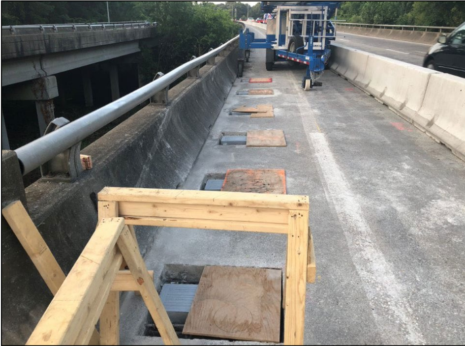
◀ Bay Avenue Installation of scupper drains
