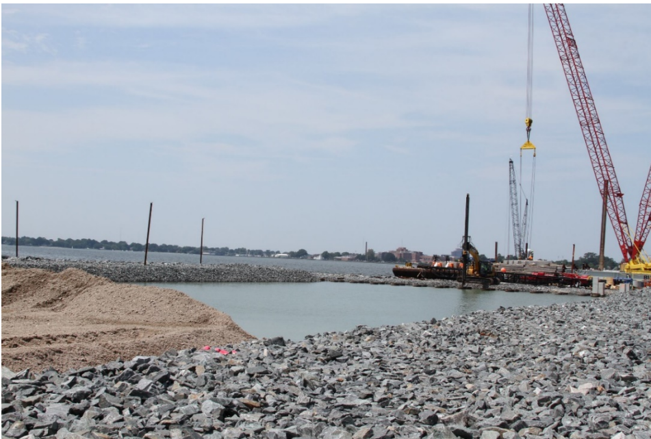
◀ North Island Expansion Last sections of fill operation.
