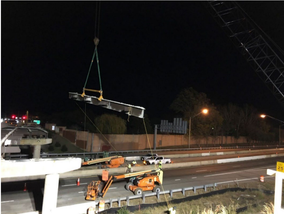
◀ Mallory St Bridge Girder Removal
