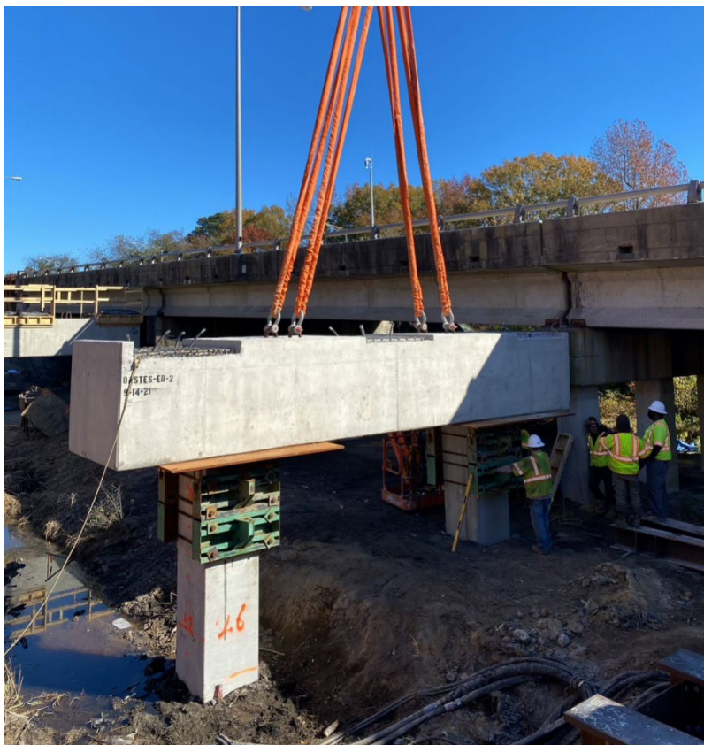
◀ Oastes Creek Bridge Precast cap placement
