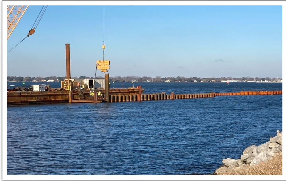
Sheet Pile Wall Separating North Island Expansion Stone from Proposed North Island Tunnel Shaft
