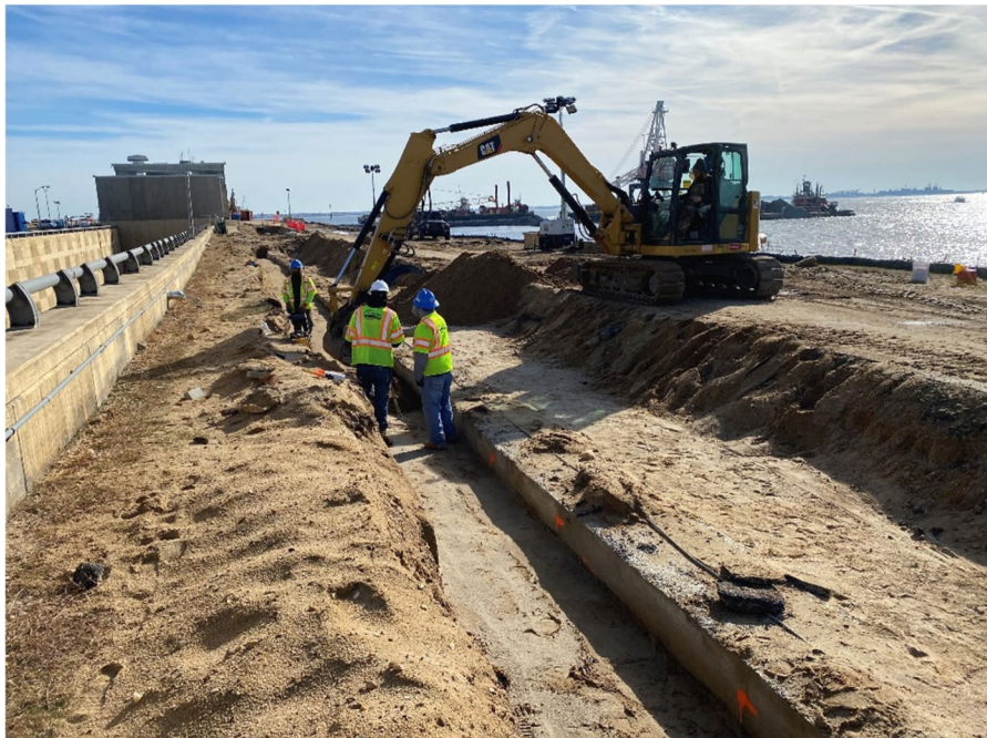
North Island Completed Medium Voltage (MV) Duct Bank Backfill
