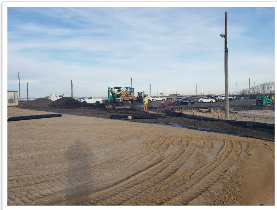
Placement of Fabric and Recycled Asphalt Material Around Office Trailer Complex at the Willoughby Staging Area
