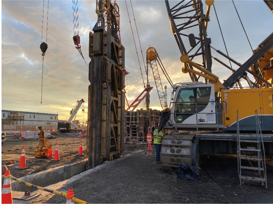
South Island Slurry Wall Hydromill Excavation
