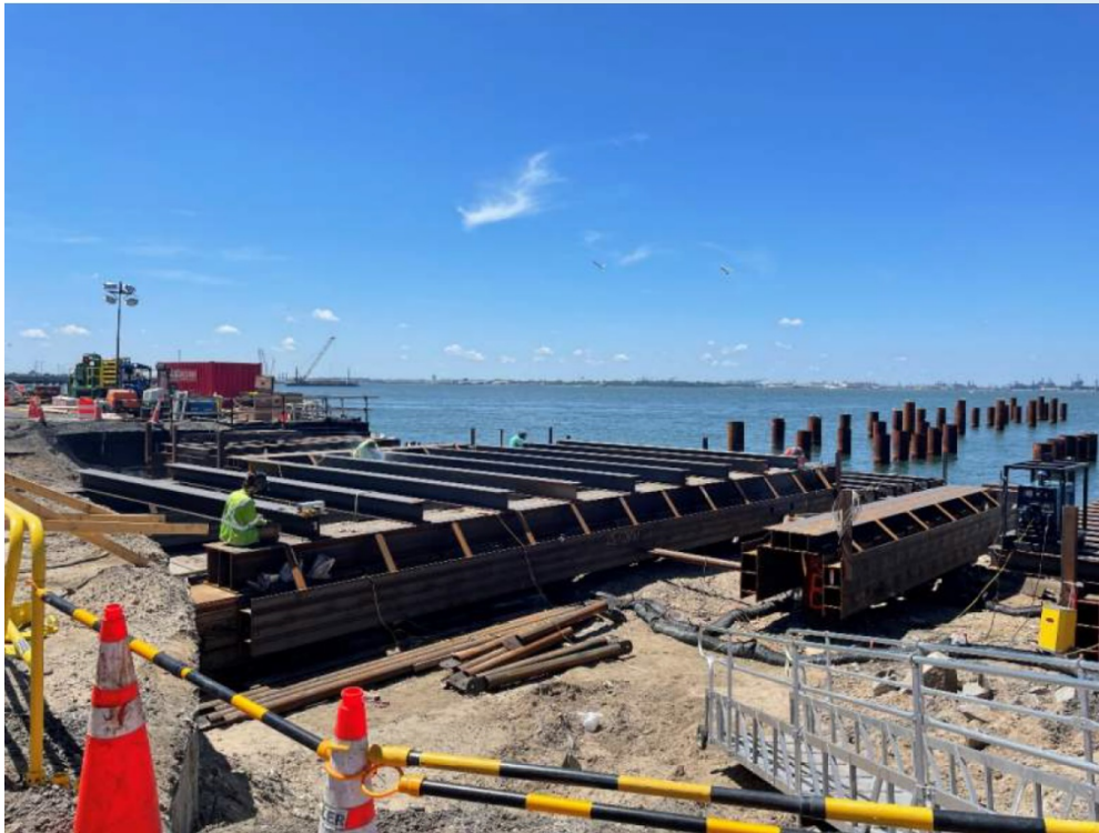
◀ South Island Sliding template fabrication for quay pile installation.
