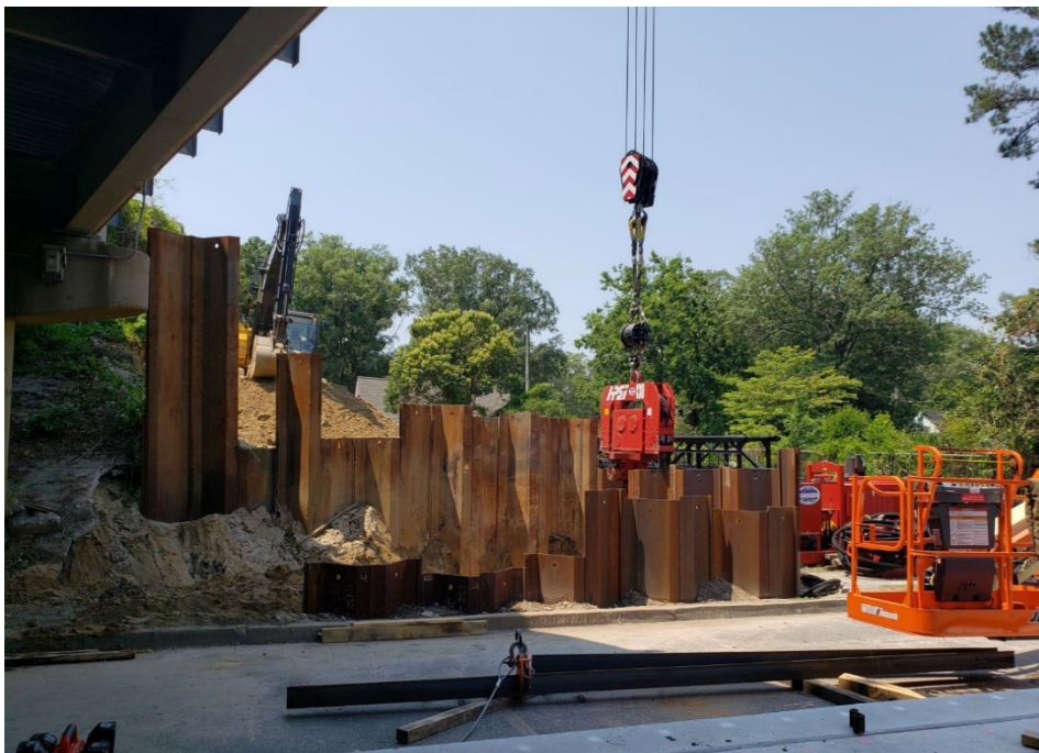
◀ Evans St Bridge Installation of cofferdam for pile foundation.
