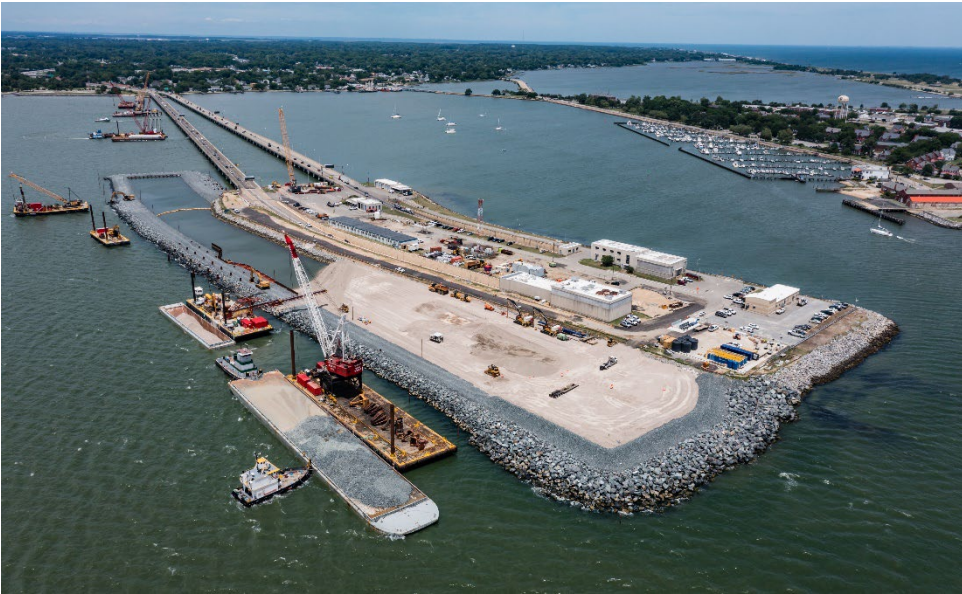
◀ North Island Expansion Fill placement progress.
