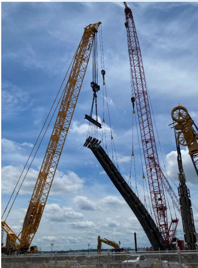
◀ South Island Tandem reinforcing cage lift for "Y" panel.
