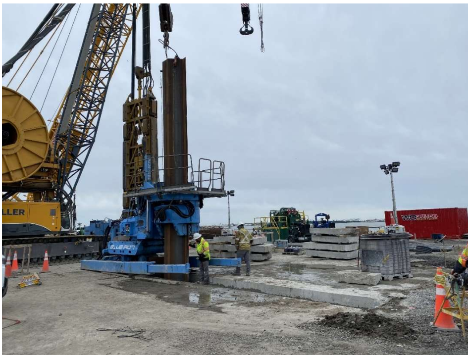
◀ South Island Installation of Sheet Piles Isolation Wall
