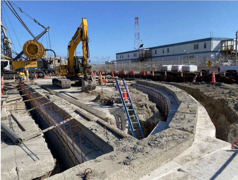
◀ South Island Guide Wall Installation for Revised Cell 2 Arch & Cross Struts
