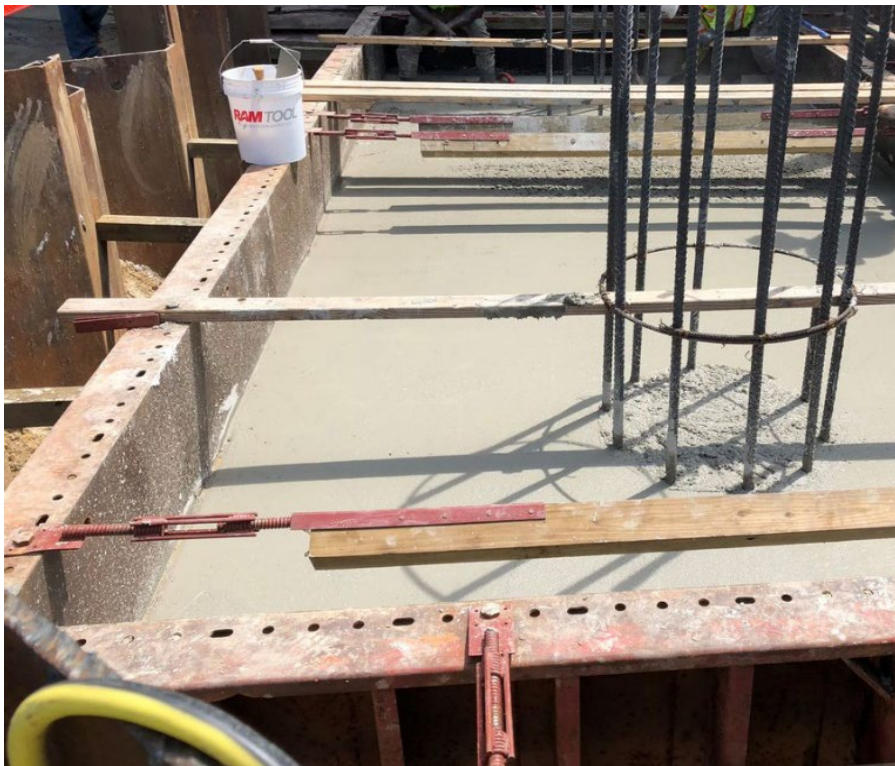
◀ Evans St Construction of footings for Piers 1 and 2.
