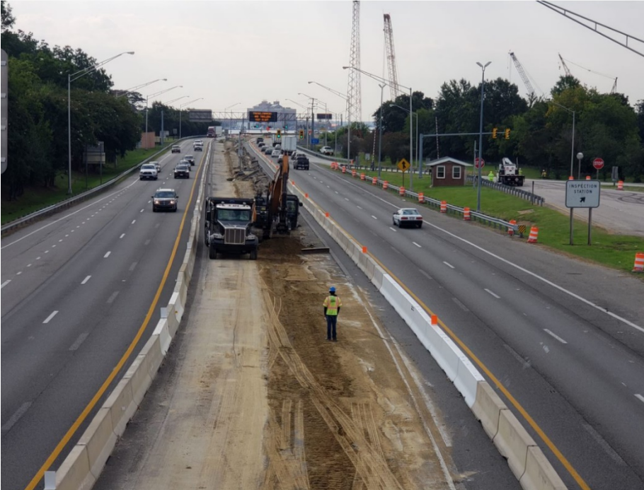
◀ Mainline I-64 - Hampton Median barrier removal.
