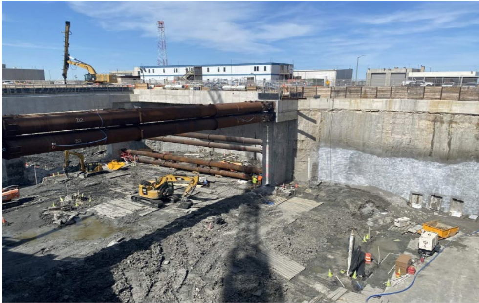
◀ South Island Cells 3 & 2 including chord strut installation
