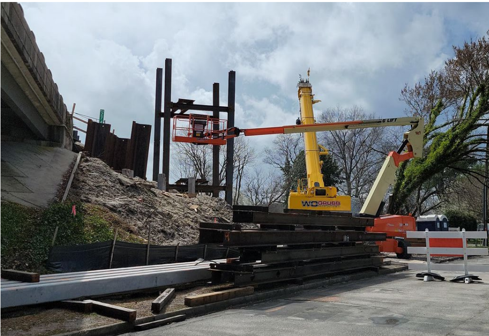
◀ Mason Creek Road Bridge Pile driving for eastbound widening.
