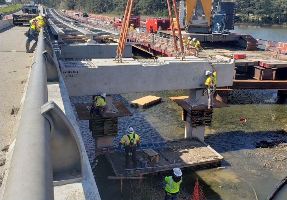
◀ Oastes Creek Bridge Setting Bent 4 precast cap for eastbound widening
