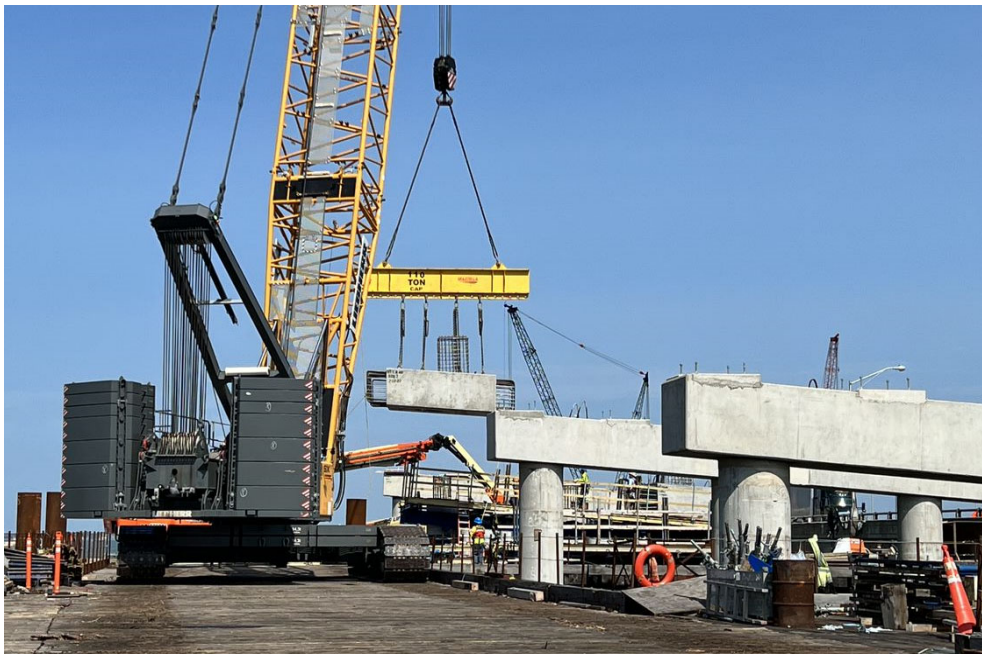
◀ South Trestle Setting of precast cap segment near Willoughby shoreline
