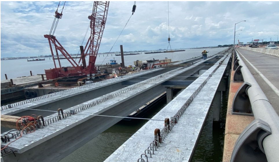
◀ Willoughby Bay Bridge Setting Span 52 girders for eastbound bridge widening
