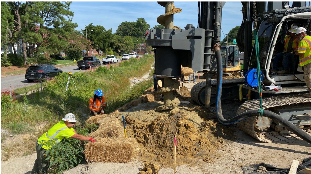
◀ I-64 EB (Norfolk) First auger-cast pile placed for sound wall
