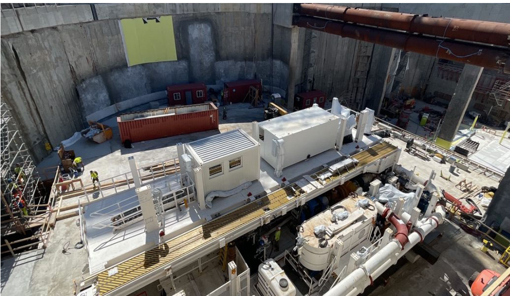
◀ South Island Assembly of TBM gantry #1, including operator's cabin
