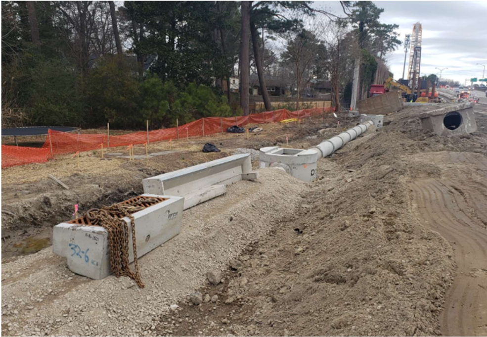
◀ Eastbound I-64 Shoulder Installing drainage in Segment 4 for the eastbound widened section
