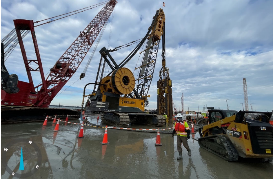
◀ North Island First slurry wall panel excavation.
