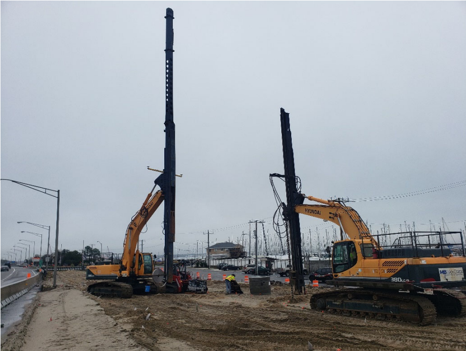
◀ I-64 EB Widening Wick drain installation for consolidation of soft soils.
