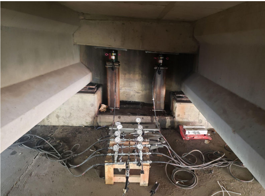
◀ Willoughby Bay Bridge Bridge jacking to support rehabilitation and bearing replacement.
