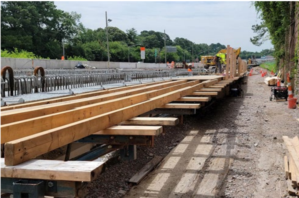
◀ Bay Ave EB Widening Installing deck overhang forms at Span 25
