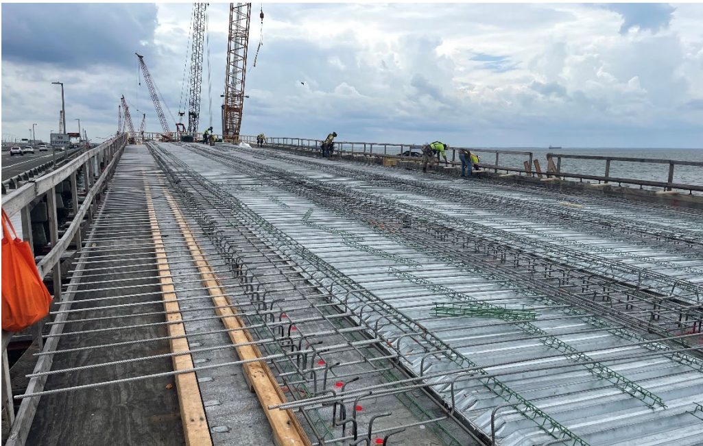
◀ North Trestle EB Rebar installation for 1 st deck placement
