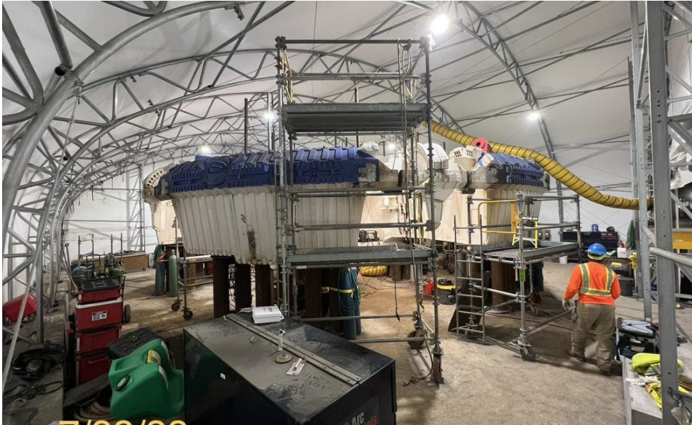
◀ South Island Inside the welding tent for the TBM cutterhead.
