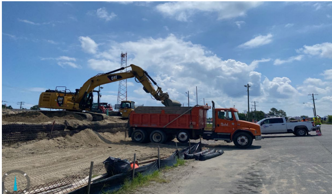
◀ I-64 EB (Norfolk) Removing temporary surcharge and wire wall from RW301 area
