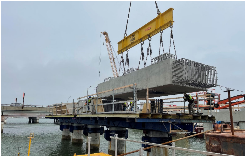
◀ North Trestle EB Cap installation
