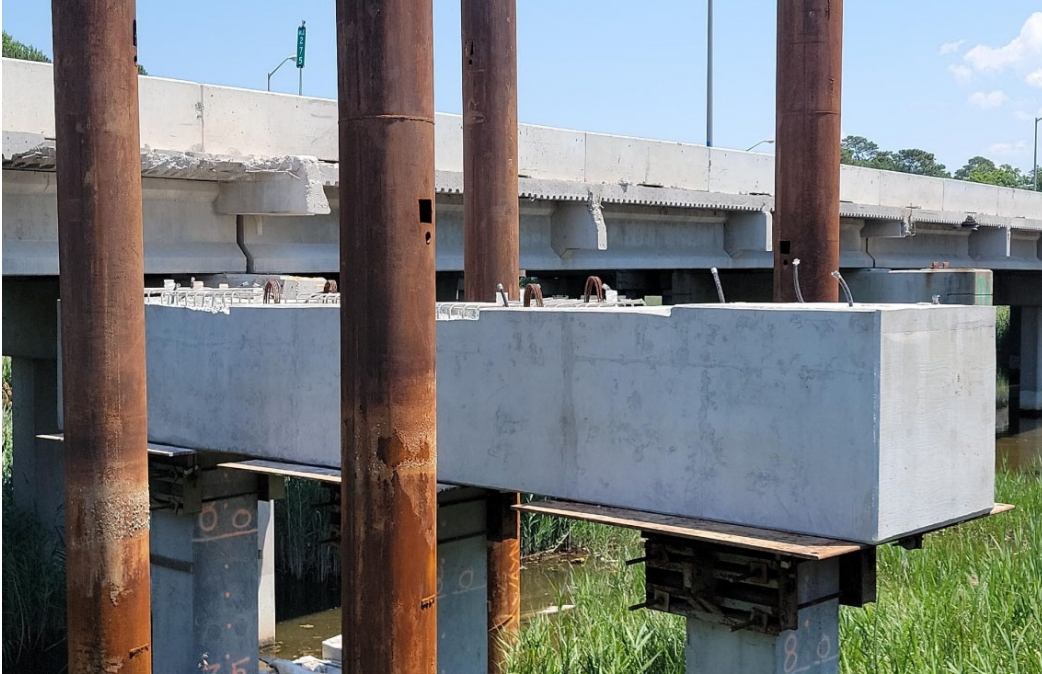
◀ Bay Avenue Bridge Installed cap at Bent 37
