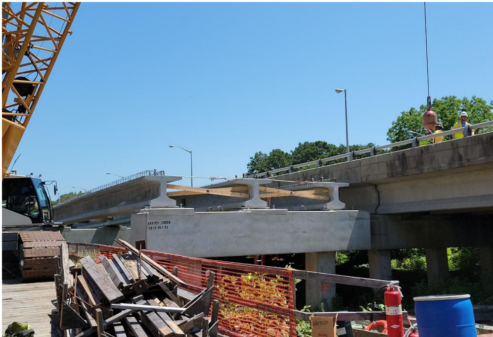
◀ Oastes Creek Cap and girder installation at Span 17
