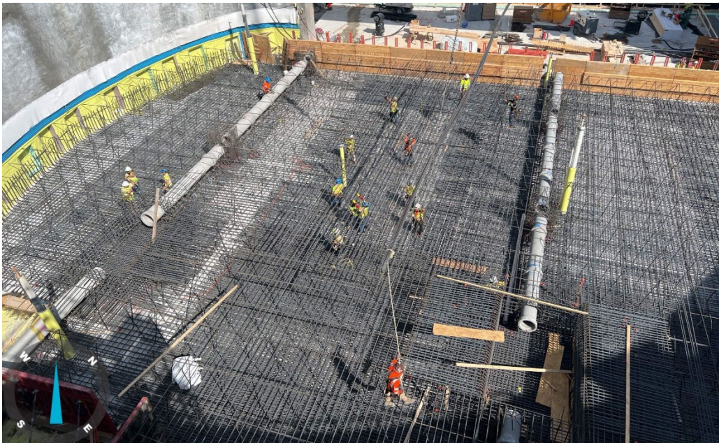
◀ South Island Reinforcing steel installation for Cell 3 base slab
