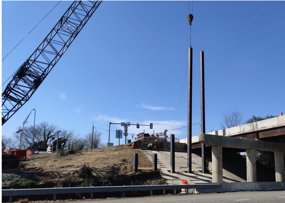
◀ Mallory St Bridge H-Pile at South Abutment for Phase 1 bridge replacement
