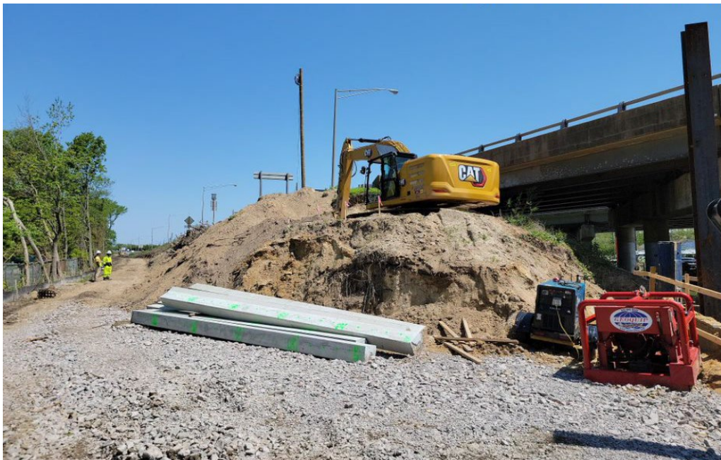
◀ I-64 EB Abutment A foundation excavation at Mason Creek Rd
