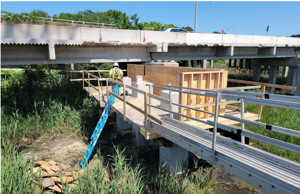
◀ Bay Avenue Bridge Installing formwork for cast-in- place cap for eastbound widening
