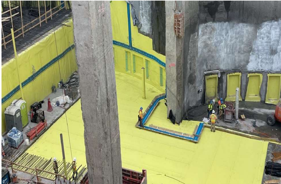
◀ South Island Waterproofing membrane installation in Cell 1 and Cell 2
