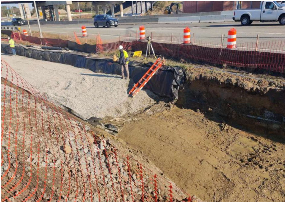
◀ I-64 EB (Segment 1) Foundation undercut at Blue Crab Substation retaining wall 02.
