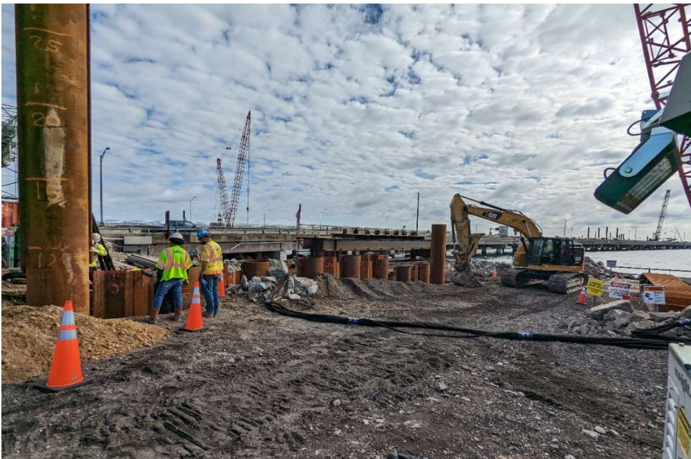
◀ South Island Expansion Cell 1 Cofferdam pipe pile installation
