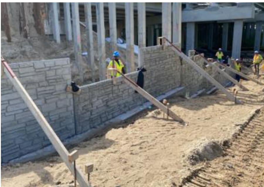
◀ Bay Avenue Retaining wall 402 panel installation
