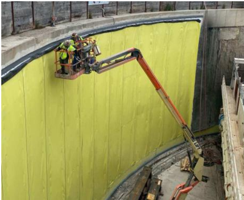
◀ South Island PVC waterproofing membrane installation in Cell 3 (west side)
