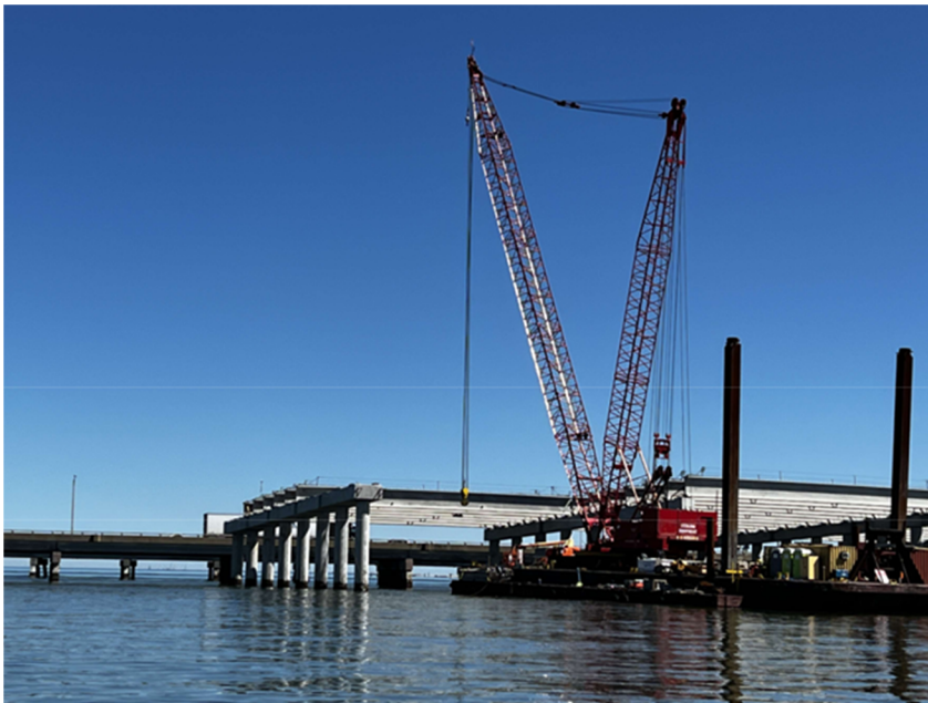
◀ South Trestle Eastbound Span 37 beam erection
