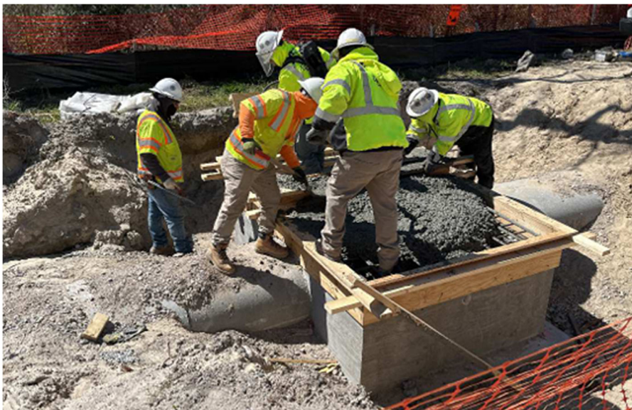
◀ I-64 EB (Segment 3) 4 th View St. ramp drainage structure installation
