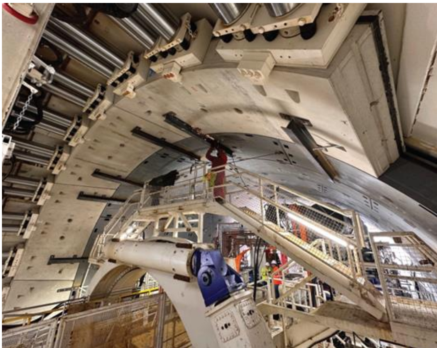
◀ HT Tunnel TBM assembling permanent ring #1
