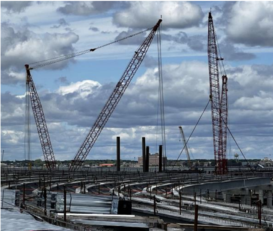
◀ South Trestle Span 28 beam erection
